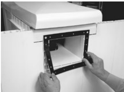
Mount the 2 adhesive seals (the first before the waterproofing is laid, the second on top of the waterproofing).
