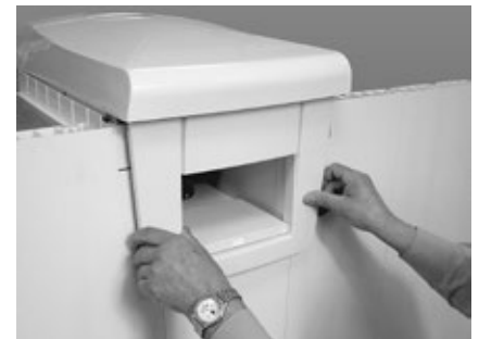
Put the trim with skimmer weir in position.
