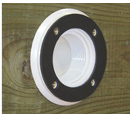
Figure 24 – Mounting the return fitting body and gasket
