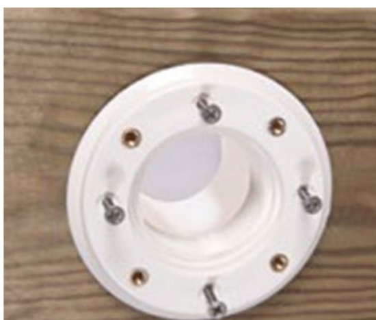
Figure 24 – Mounting the return fitting body and gasket
