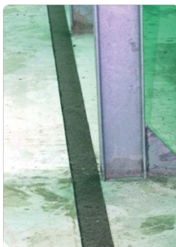
Figure 7 – Laying the bituminous strips
