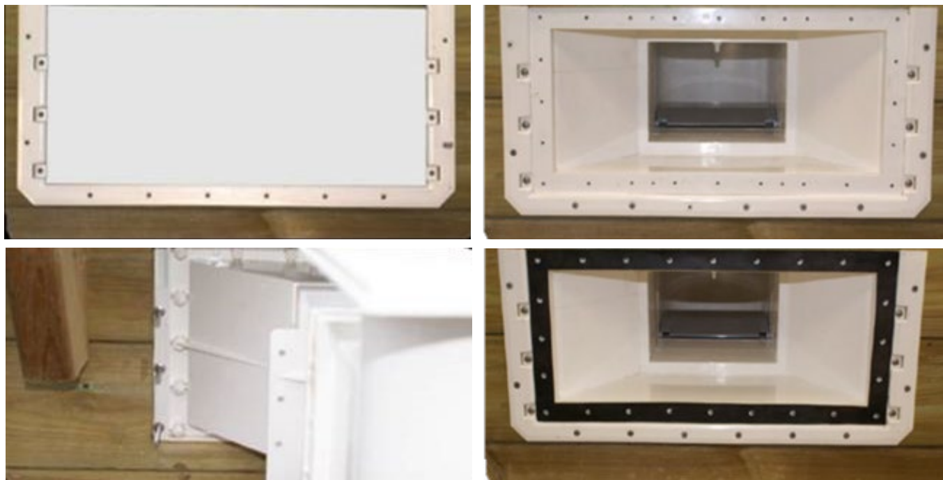
Figure 24 – Montage du skimmer
