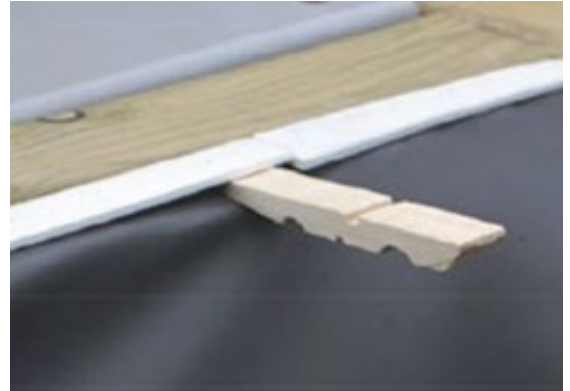
Figure 33 – Blocking the liner in position using half clothes pegs
