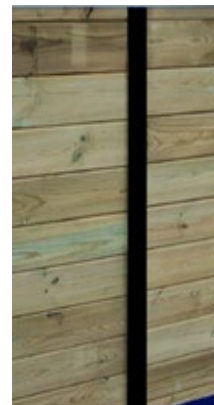
Figure 22 – Protective adhesive strip
