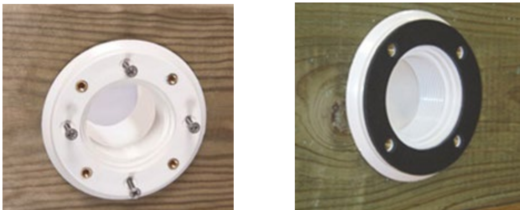
Figure 26 – Mounting the return fitting body and gasket
