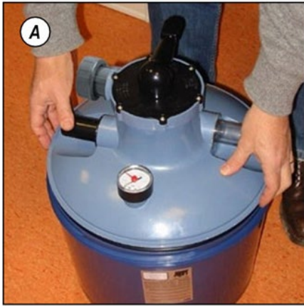
Hold the lid over the filter tank.
