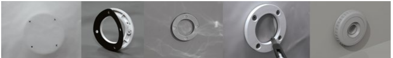
Figure 36 – Installing the return fitting flange
