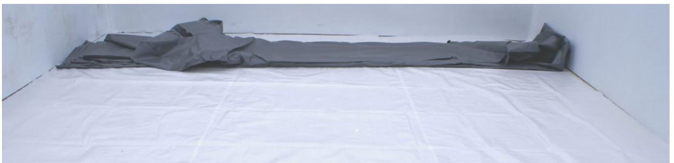
Figure 34 – Unfolding the liner
