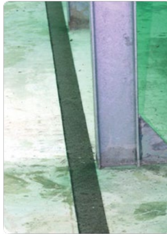
Figure 6 – Laying the bituminous strips
