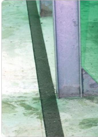
Figure 8 – Laying the bituminous strips
