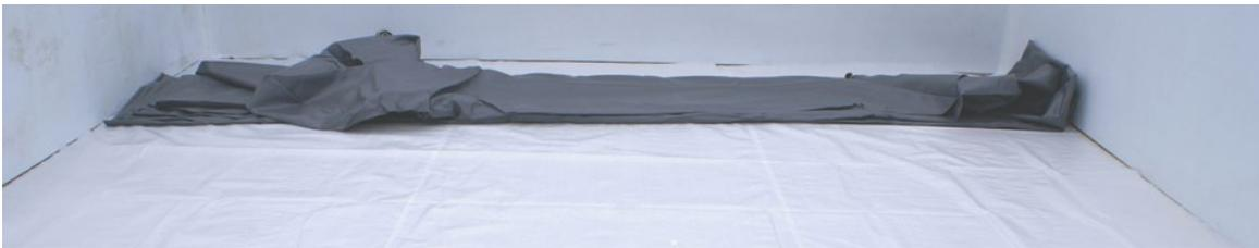
Figure 33 – Unfolding the liner
