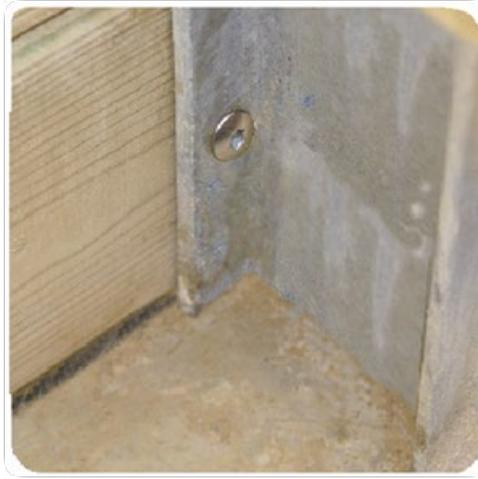
Figure 11 – Fastening the slats to the supporting braces
