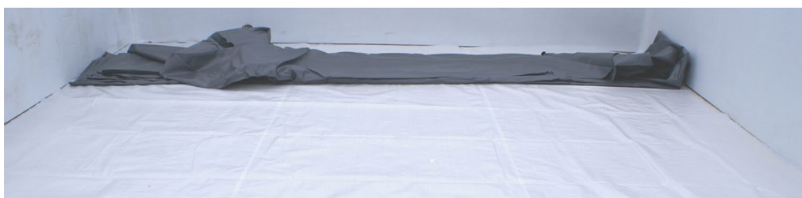
Figure 33 – Despliegue del liner
