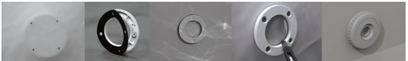
Figure 35 – Installing the return fitting flange
