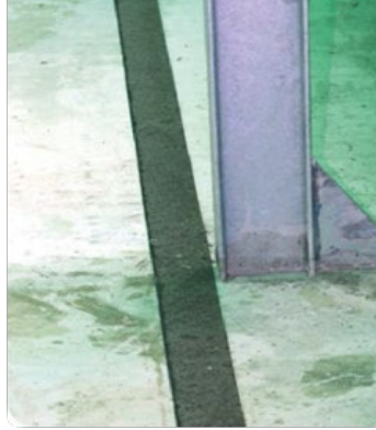
Figure 8 – Laying the bituminous strips
