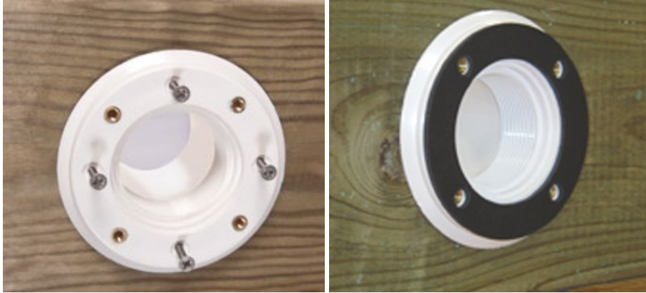
Figure 24 – Mounting the return fitting body and gasket
