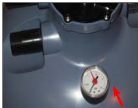
Position the pressure gauge correctly and place it in its housing.
