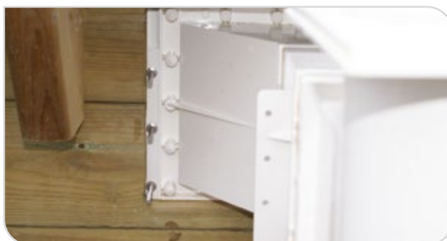
Figure 34 – Verouillage du skimmer
