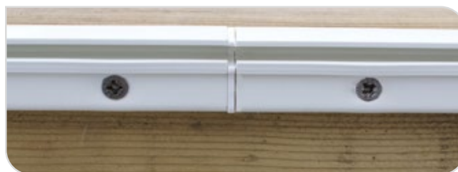
Figure 29 – Liner locking track
