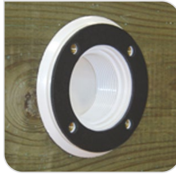
Figure 38 – Applying the gasket
