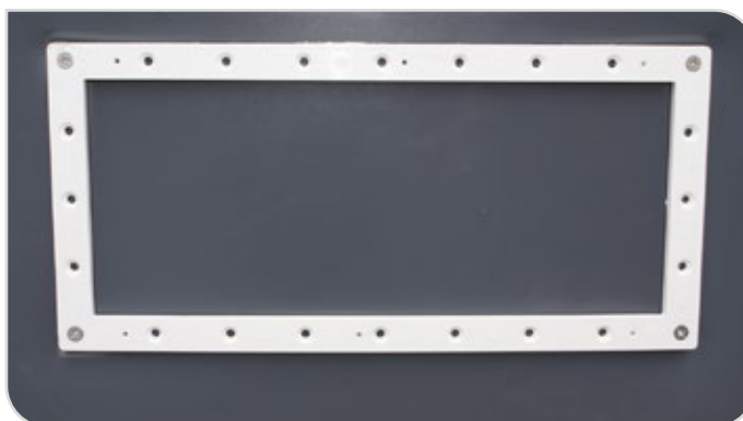
Figure 52 – Mount the second flange
