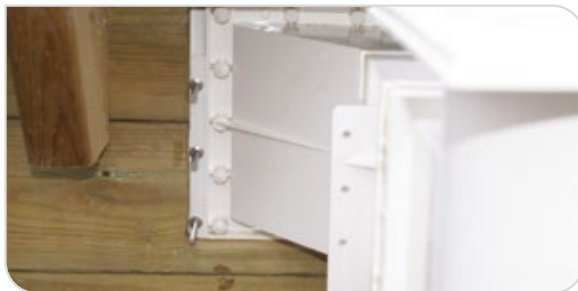
fasten the skimmer in position
