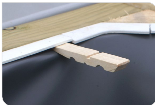
Figure 41 – Hold the liner in position with half logs
