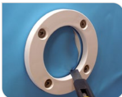
Figure 53 – Cut out the liner
