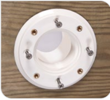
Figure 37 – Screwing the body in position
