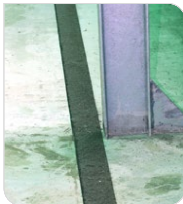
Figure 15 – unrolling the asphalt strips
