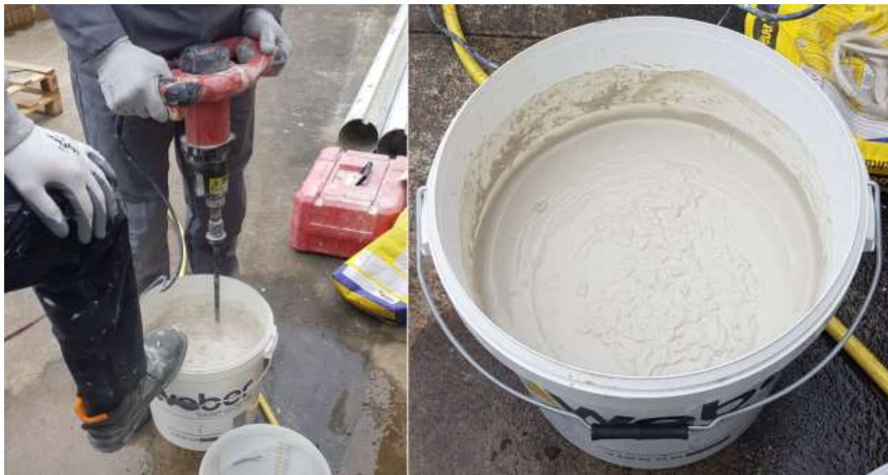
Figure 36: Mixing the sealant
